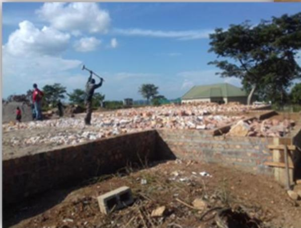
It has requires 18 trips of hard rock to level up the foundation and to make it ready for concrete slab.
