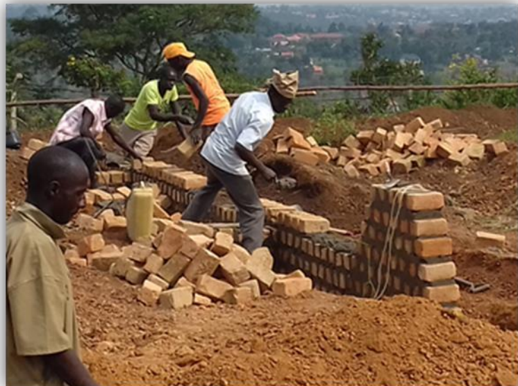
By the beginning of last week, the brick laying for the foundation was all done.
