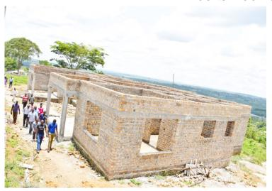
As of June – July, construction of the first residential facility at the PT Center had been built up to the wall-plate and ready for the roof.
